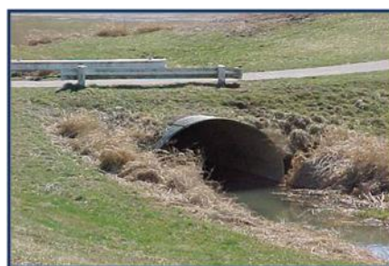
Before Mitigation and After Mitigation
